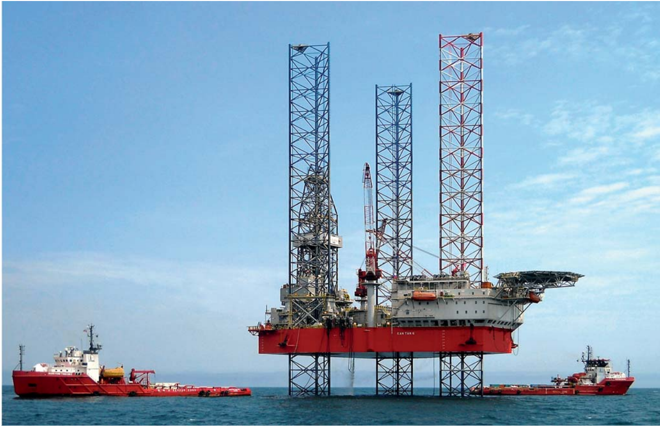
Jack-up drilling rig at Veninsky block, Sakhalin-3 project
