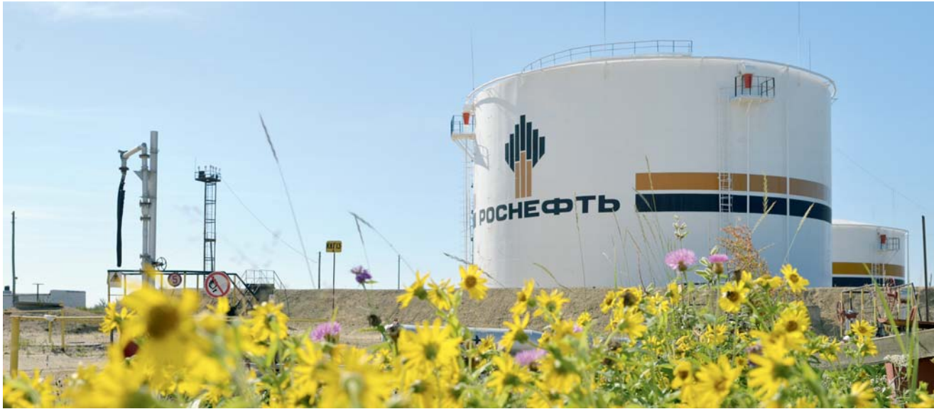
Tank farm of Sakhalinmorneftegaz
