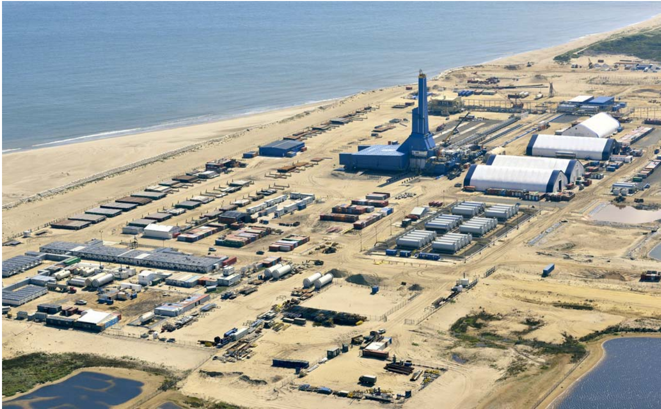
Drilling unit «Yastreba» at Chaivo field, Sakhalin-1 project
