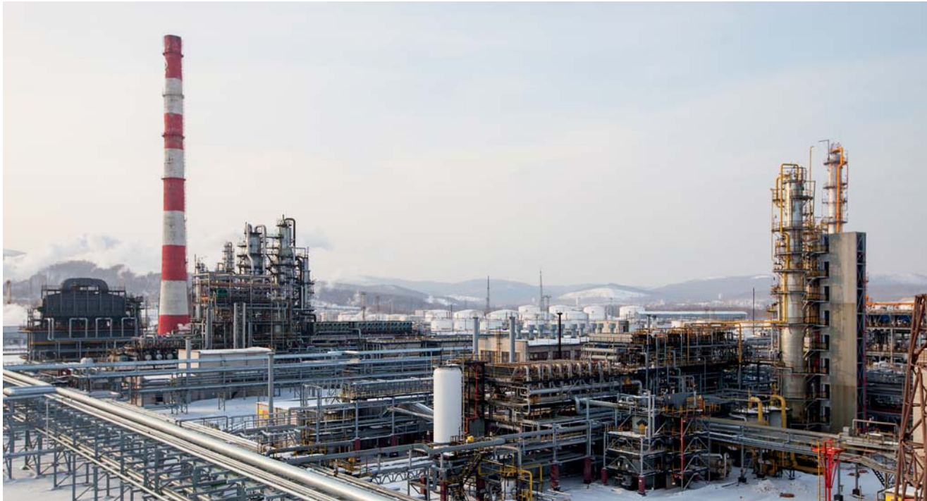
Reforming unit at Komsomolsk refinery
